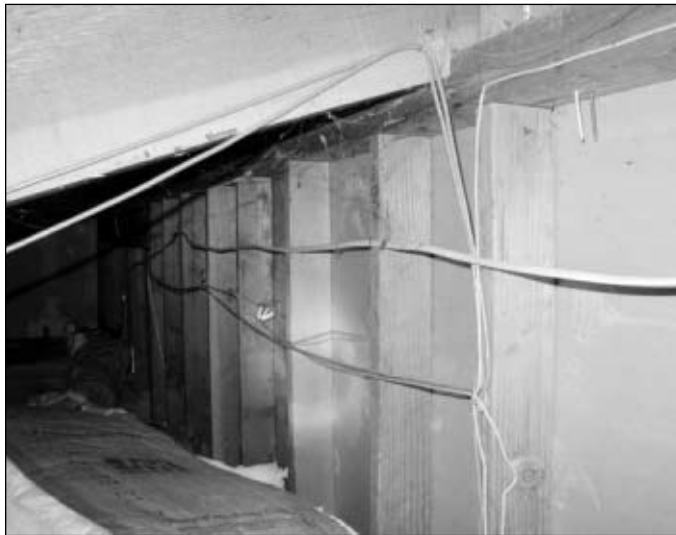
Kneewalls like this one are often found to be uninsulated—a major deficiency.
