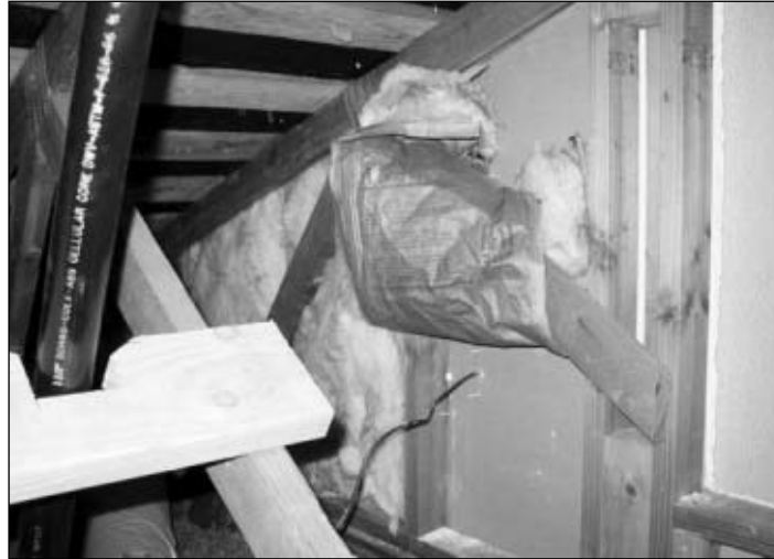
Home inspections often reveal insulation failures caused by other trades—in this case a cable installer.
