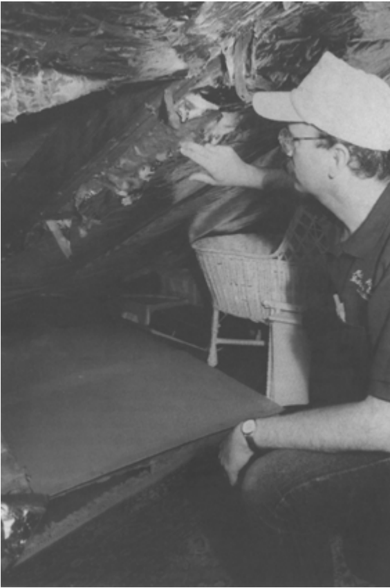
During field training, Joe Kuonen shows contractors discolored attic insulation, an indication of unwanted airflow.
